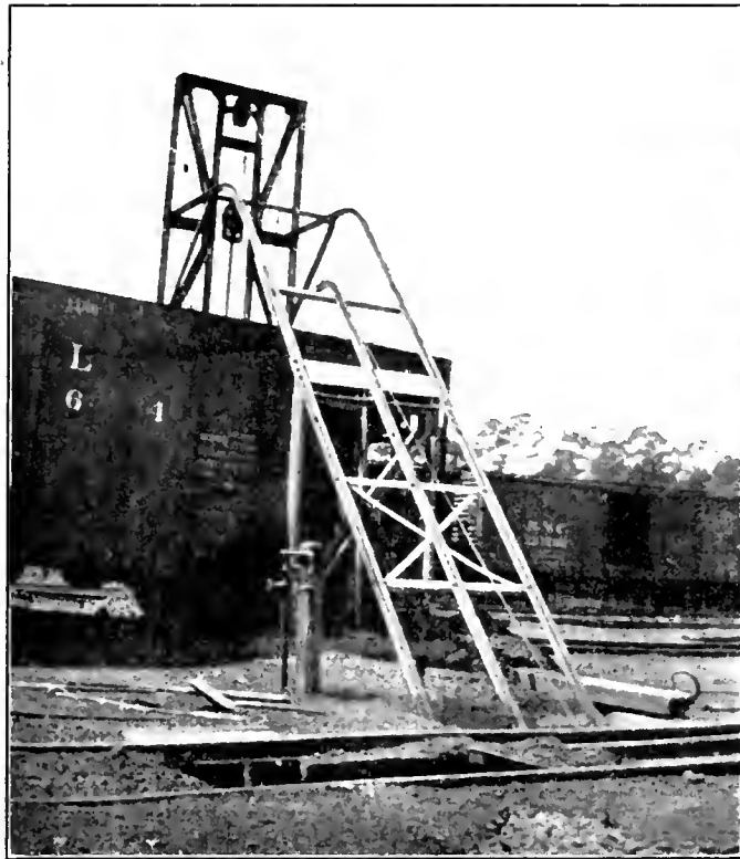
Loading Cinders from Locomotive Ash Pits
